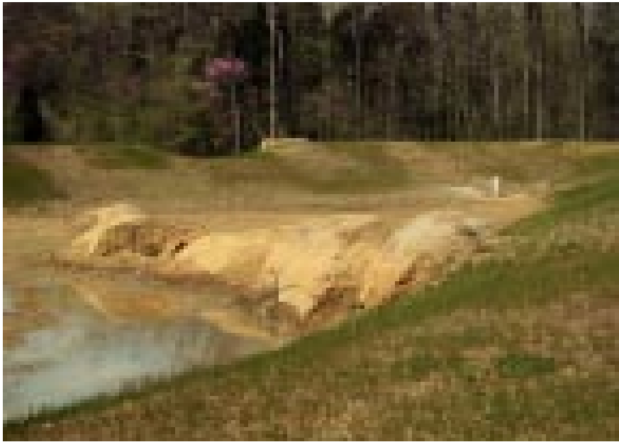
Final stages of pond construction with emergency spillway.
