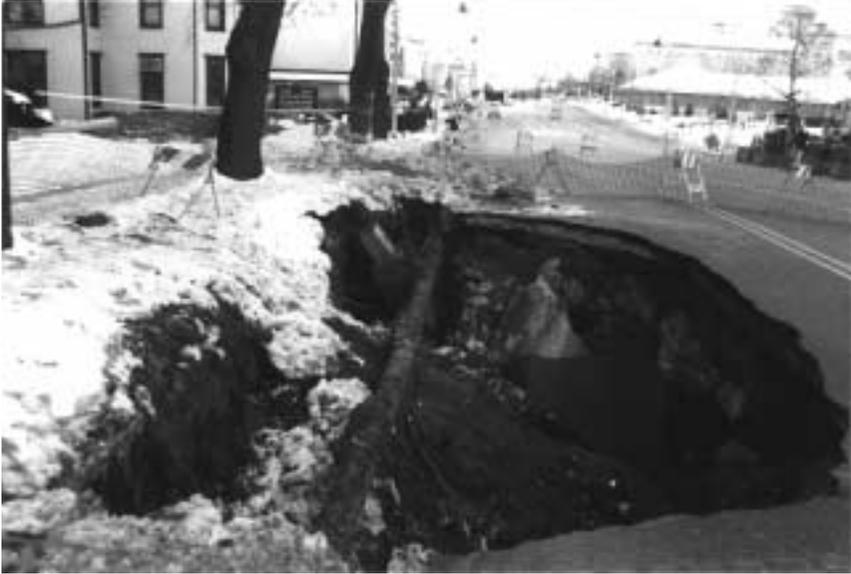
**Figure 12.** This sinkhole in Dauphin County has exposed a utility pipeline.
