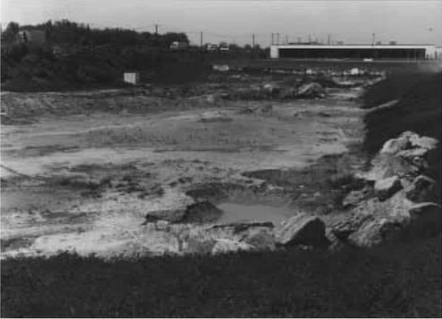
**Figure 16. Sinkholes in a storm-water retention basin along U.S. Route 22 in Lehigh County.**
