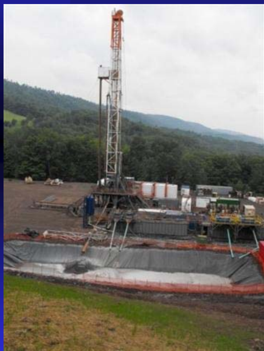
Site Development (Switching to Closed Loop Drilling)
